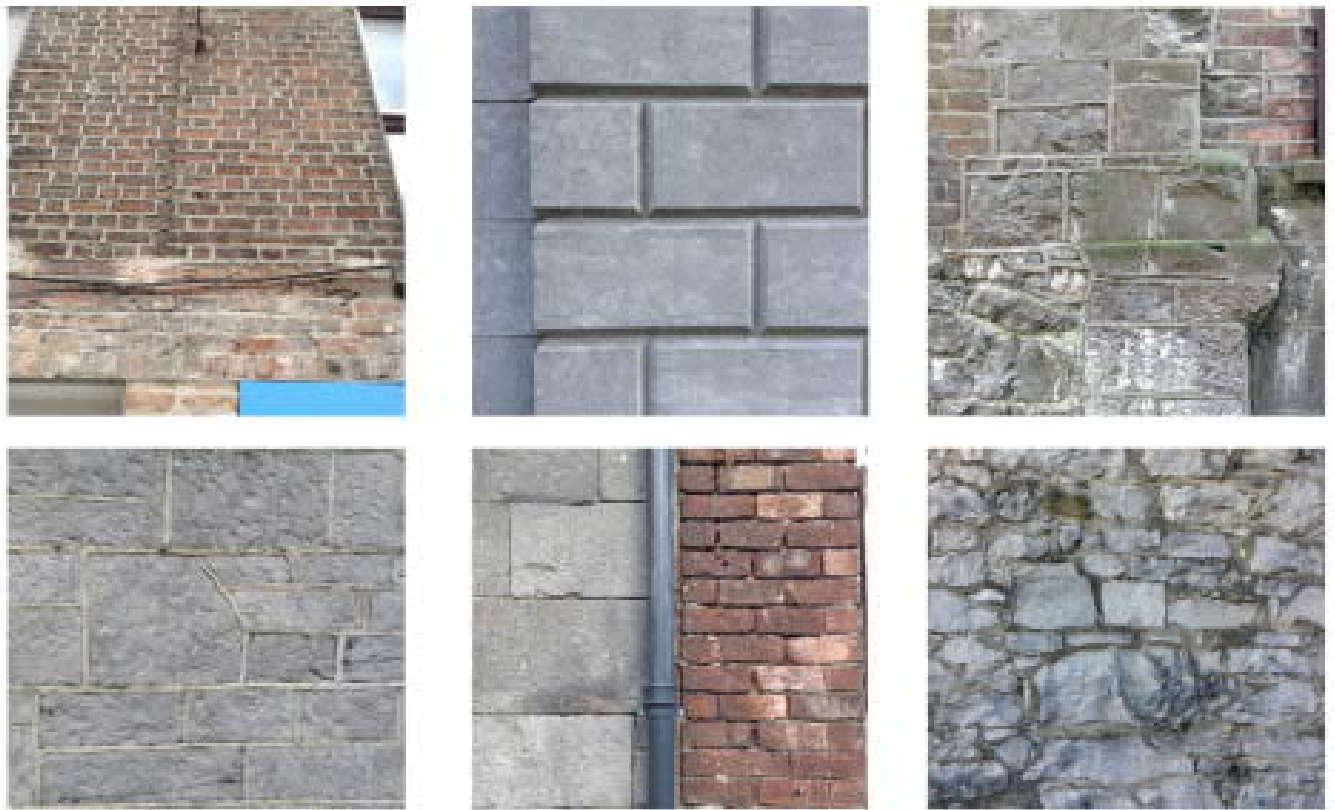
Figure 7.01 Existing Materials Palette
