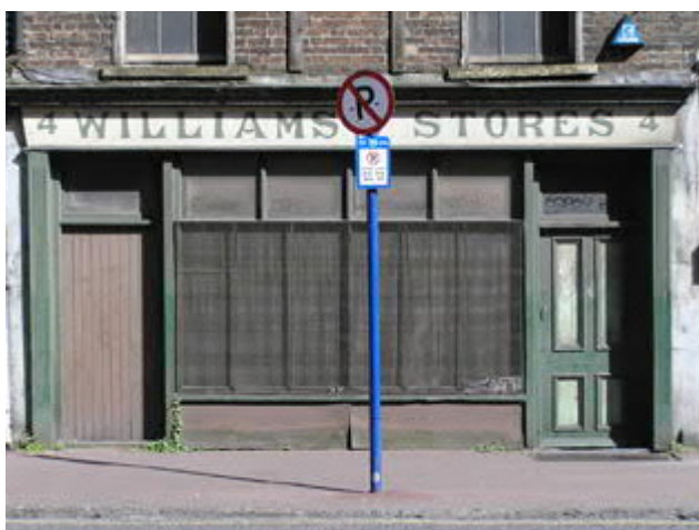
Figure 4.03 4 Patrick Street : Timber shopfront at ground floor level, c. 1880.
